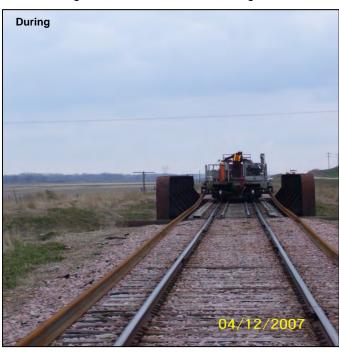
A & K Railroad Materials is shown distributing the continuously welded rail near Akron, IA.
