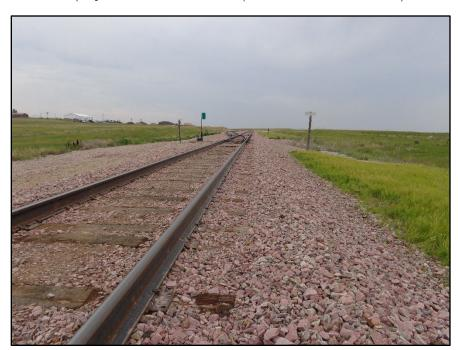
With a \$978,200 CRISI grant, ASLRRA member Rapid City, Pierre & Eastern Railroad was able to make significant upgrades to its 100-year-old track. This photo from RCPE shows a section of the two-and-a-half mile project: a new turnout and some new 115-pound continuous welded rail.
