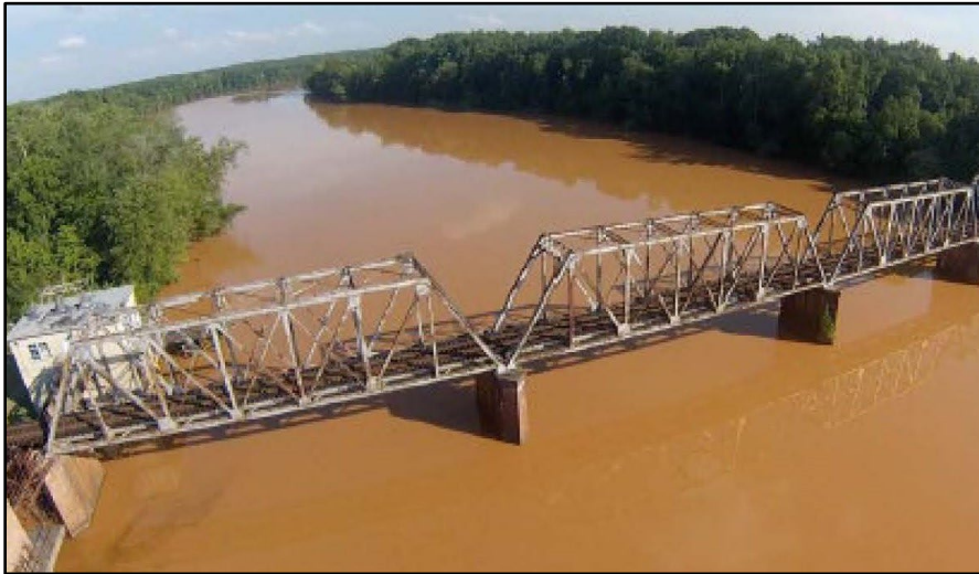
ASLRRRA member L&C Railroad used funding from a CRISI grant to upgrade the Catawba River Bridge (above) to handle 286,000-pound cars at Class II train speeds. L&C was also able to purchase three new locomotives (below) with CRISI funding.
