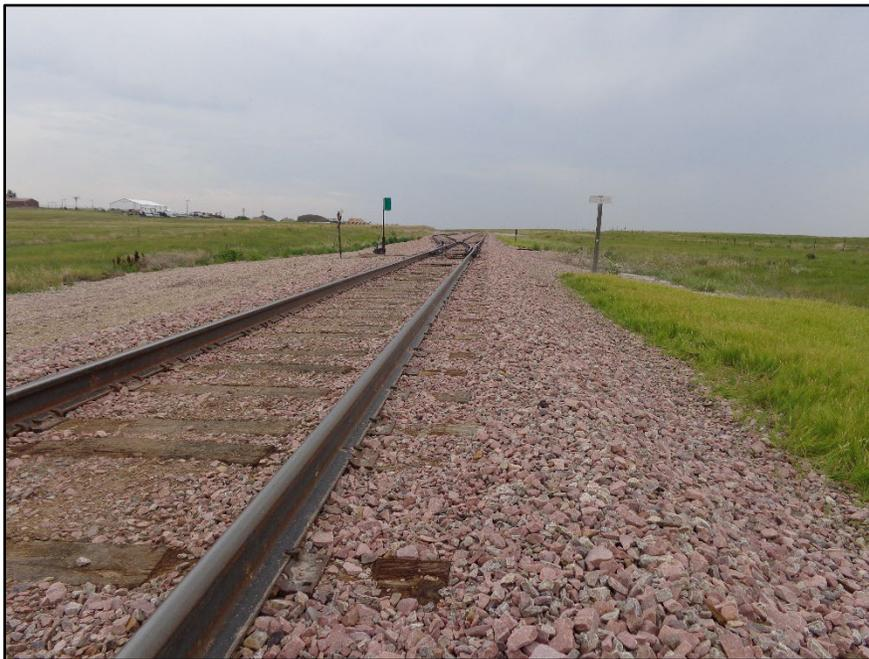
With a \$978,200 CRISI grant, ASLRRRA member Rapid City, Pierre & Eastern Railroad was able to make significant upgrades to its 100-year-old track. This photo from RCPE shows a section of the two-and-a-half mile project: a new turnout and some new 115-pound continuous welded rail.
