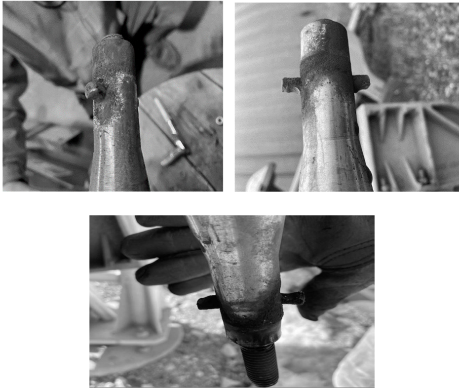
Figures 4,5,6-Heavily oxidized and worn king pin tabs
