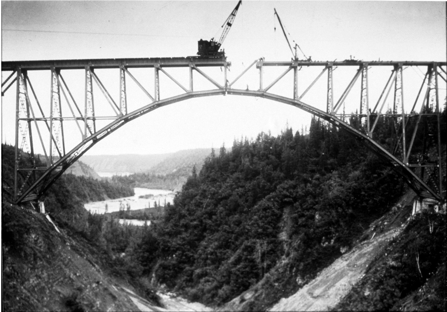
Hurricane Gulch Bridge completed in 1921
